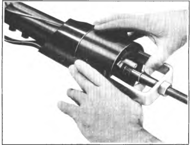
Fig. 3B4-30--Installing Snap Ring
