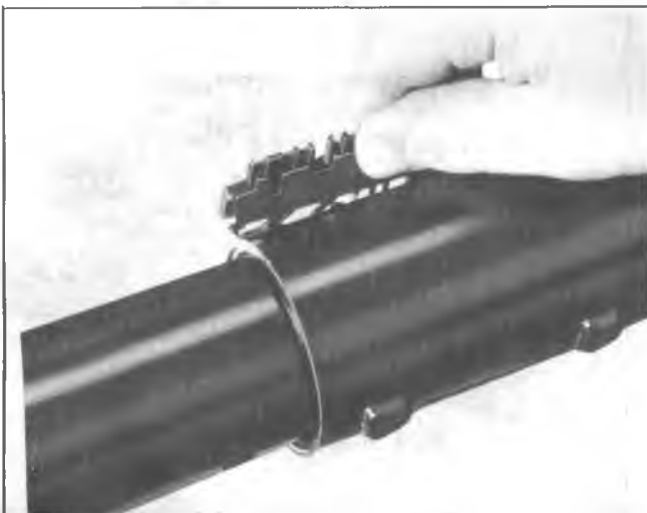
Fig. 3B4-29--Installing Switch Connector Onto Jacket Clips
