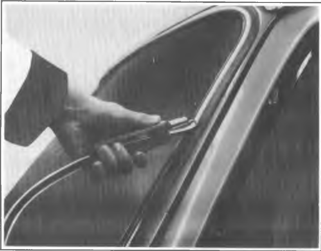
Fig. 2D-19--Installing Reveal Molding
