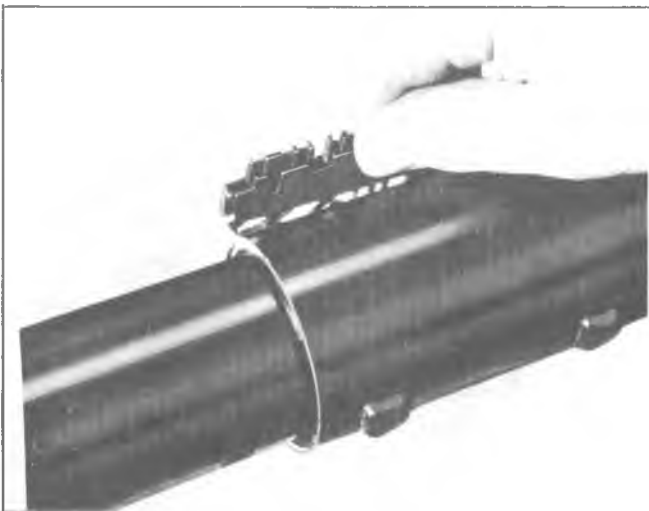
Fig. 3B4-29--Installing Switch Connector Onto Jacket Clips
