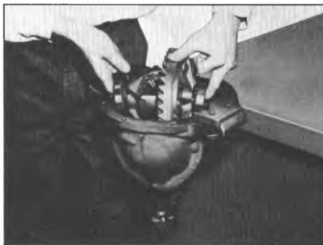
Fig. 8C—Installing Differential Assembly
