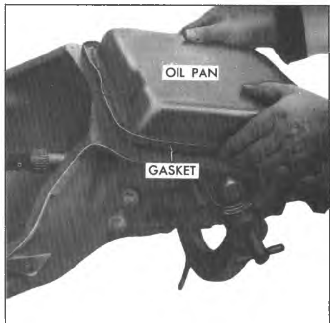
Fig. 9N--Removing Transmission Oil Pan
