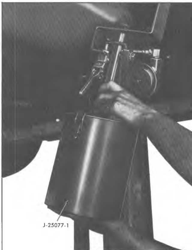
Fig. 7—Installing Vibrator
